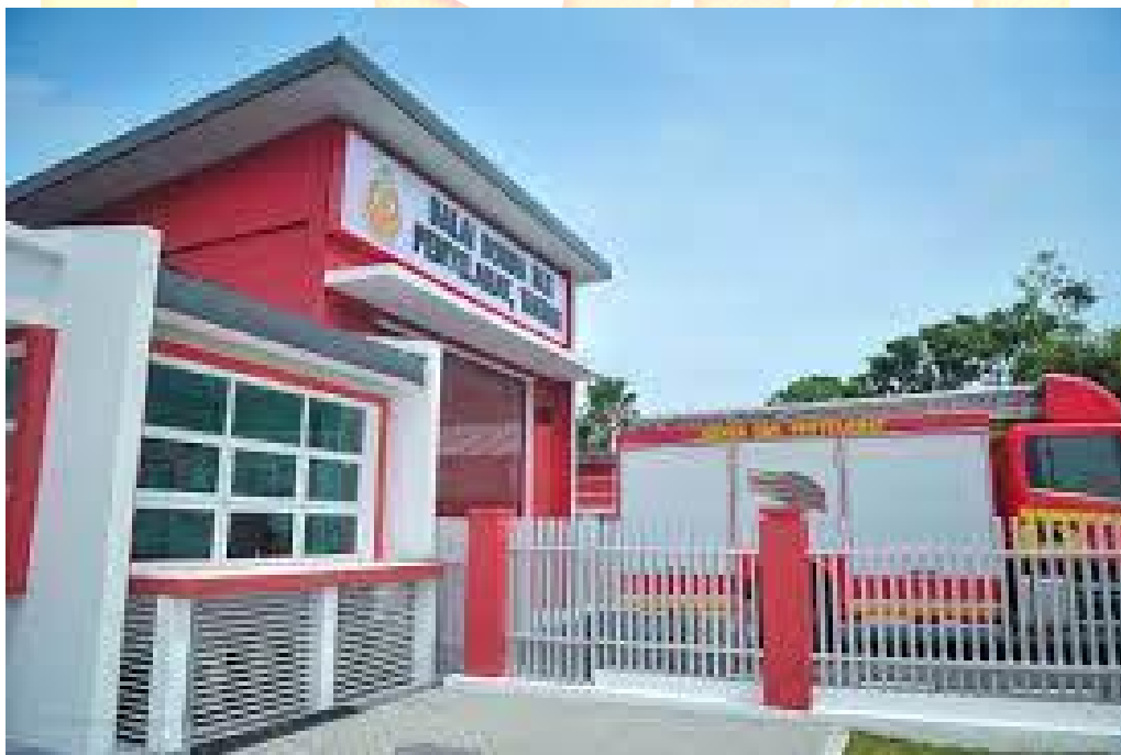
Figure 2: Fencing surrounding the facility
